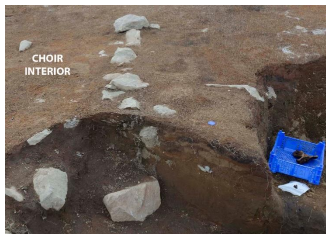
Figure 21. Cross section of the church wall in the northeast corner of the choir, exposed by the electrical trench originally dug by RARIK. View to the west.
